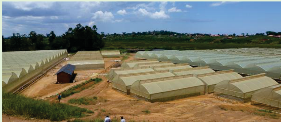
MULTISPAN 960 FIXED OPEN VENT | 25 HA | ROSES | UGANDA
