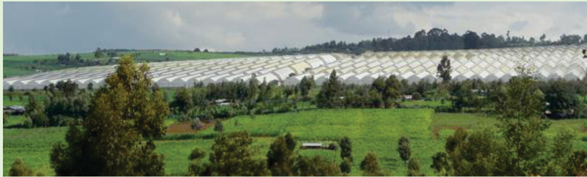
MULTISPAN 960 FIXED OPEN VENT | 40 HA | ROSES | KENYA
