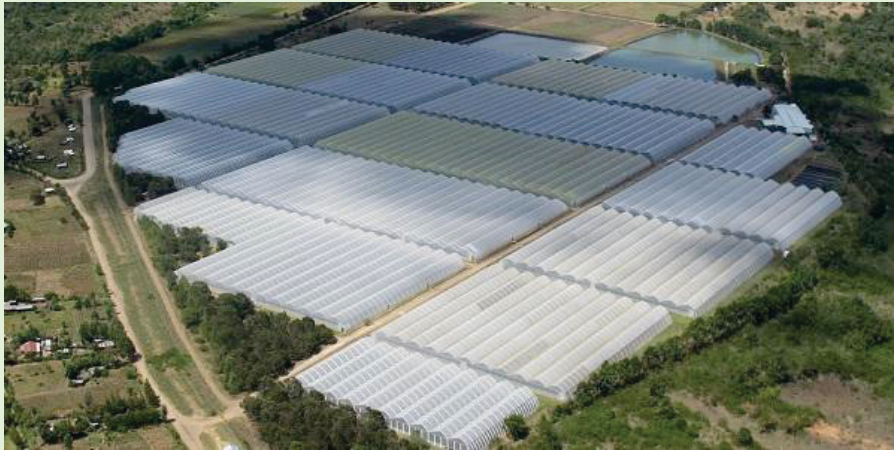
MULTISPAN 960 FIXED OPEN VENT | 22HA | ROSES | KENYA
